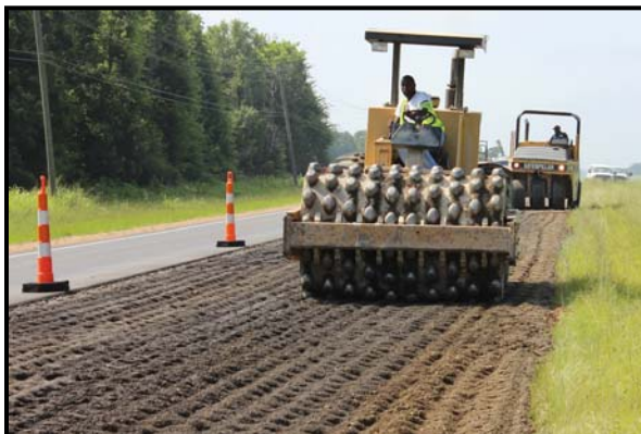
e) CP-563C Compaction (Background: PS-360C)
