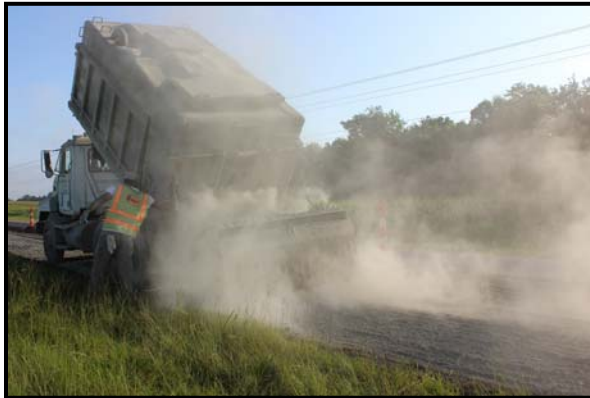
a) Cement Spreading
