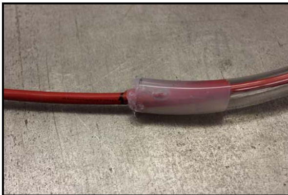
e) Silicone Seal at End of Flex Tubing
