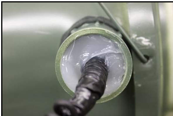
e) Sealed Temperature and Humidity Cables
