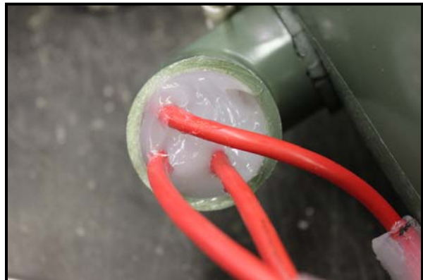
d) GS3 Cables Sealed with Silicone
