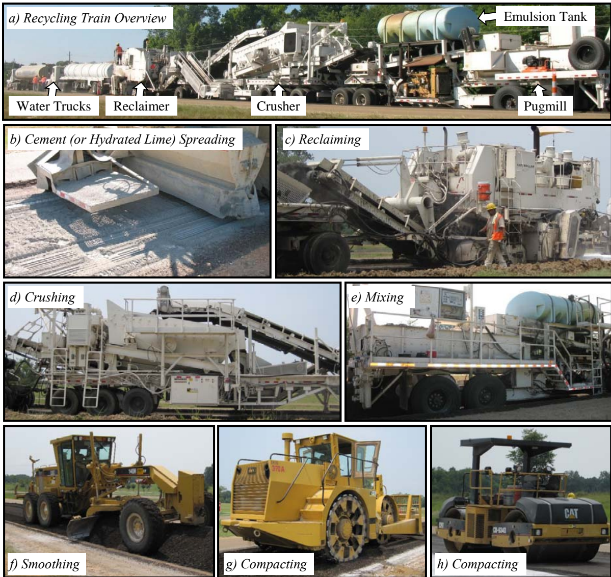
Figure 5.2. US-49 CIR Construction Photos
