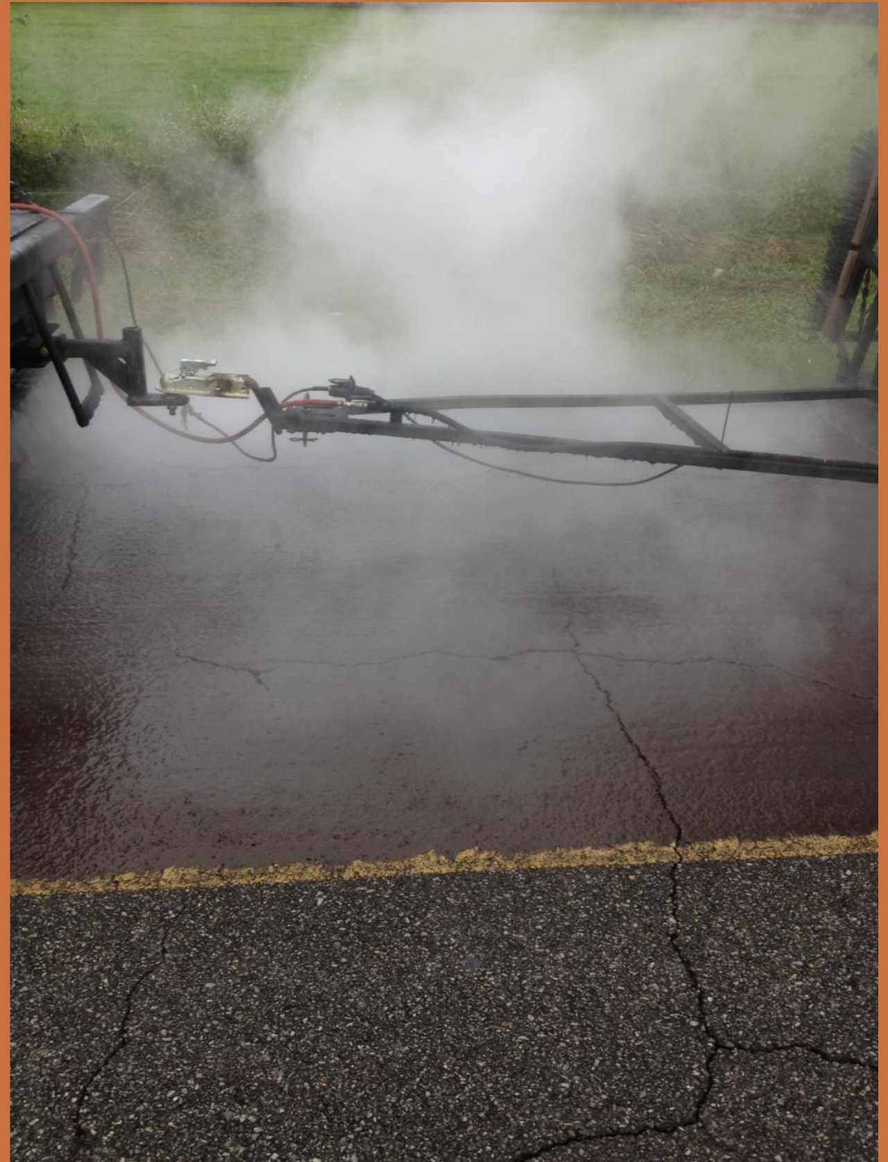
After Emulsion is Sprayed
