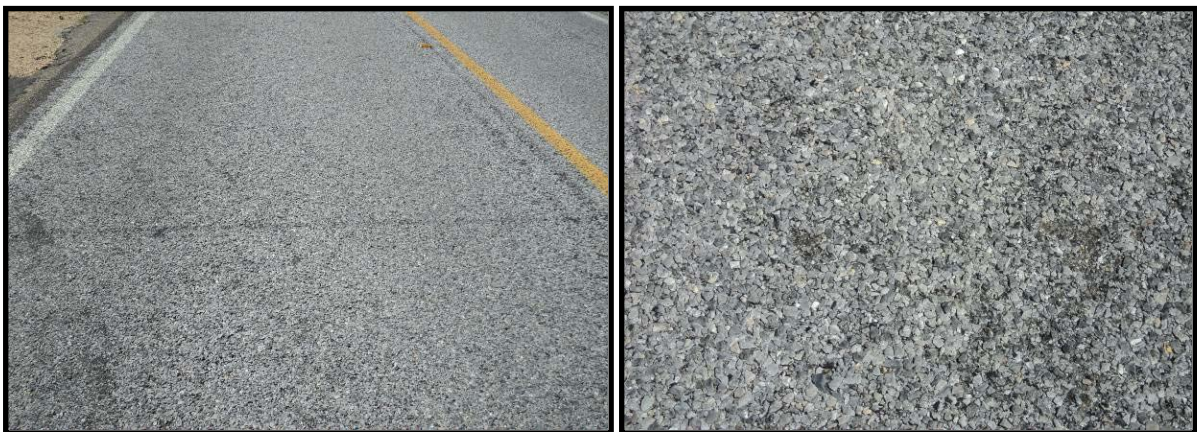
Figure 5.11. Hwy 44 Section 2 Intermediate Survey (09/10/2012)
