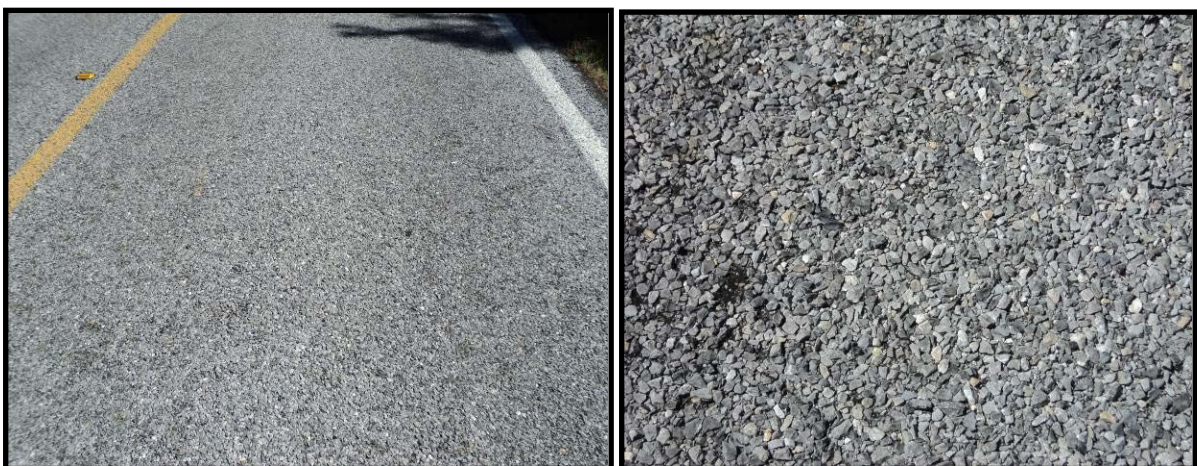
Figure 5.12. Hwy 44 Section 3 Intermediate Survey (09/10/2012)
