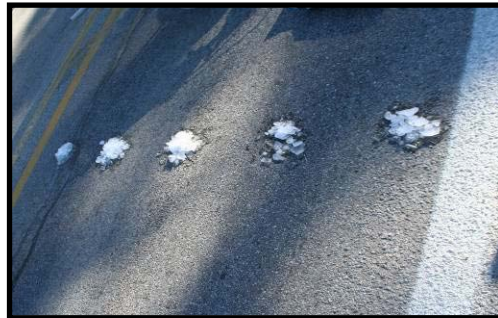
Figure 5.23. Pre-Marked Locations With Ice Prior to Coring
