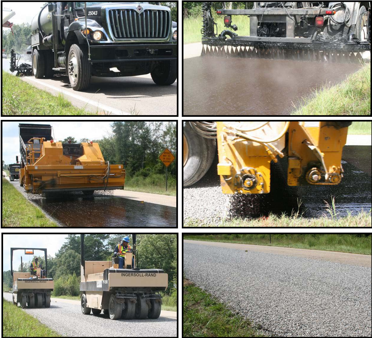
Figure 5.7. Hwy 44 Chip Seal Application (09/20/2011)
