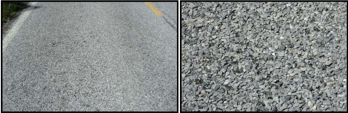
Figure 5.10. Hwy 44 Section 1 Intermediate Survey (09/10/2012)
