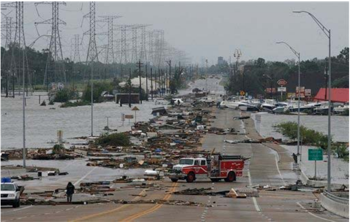
Figure 4: Debris Making Road Near Impassable
