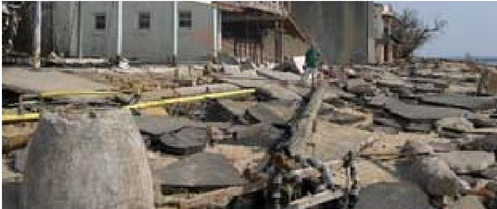
Figure 10: Example of Severely-Damaged from Damaged-Dangerous Category
