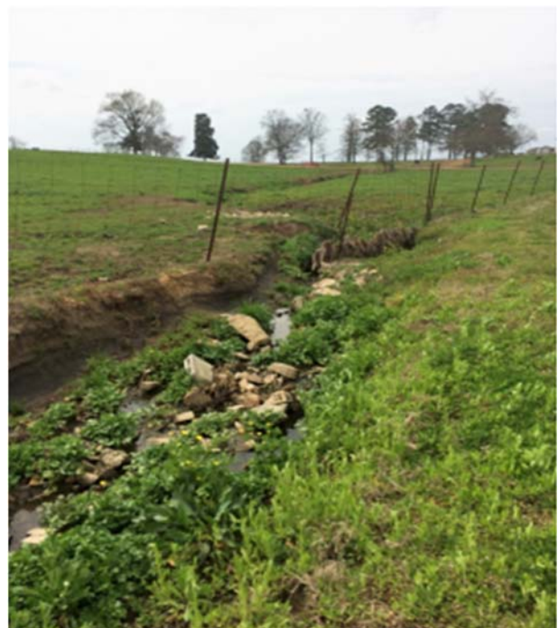
Site 7d NRCS Practice 410 – Grade Stabilization Structure (Check Dam)
