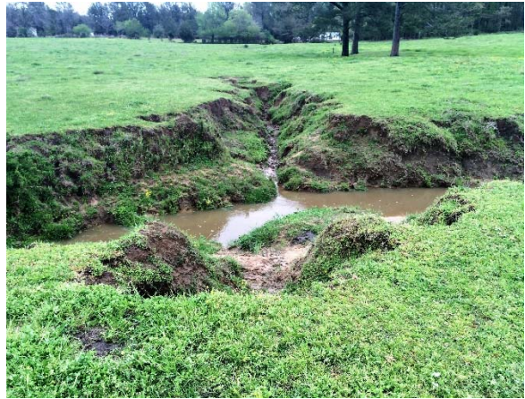
Site 13a East Side of Creek NRCS Practice 382– Fencing
