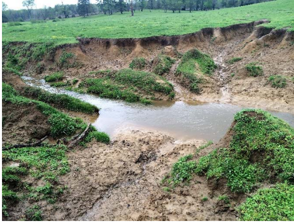
Site 15a NRCS Practice 578 – Stream Crossing
