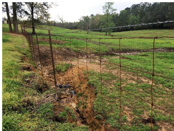
Site 12a NRCS Practice 410 – Grade Stabilization Structure (Check Dams)
