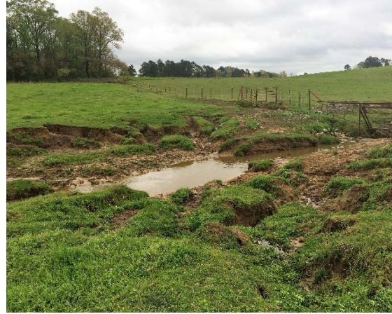
Site 15b NRCS Practice 578– Stream Crossing
