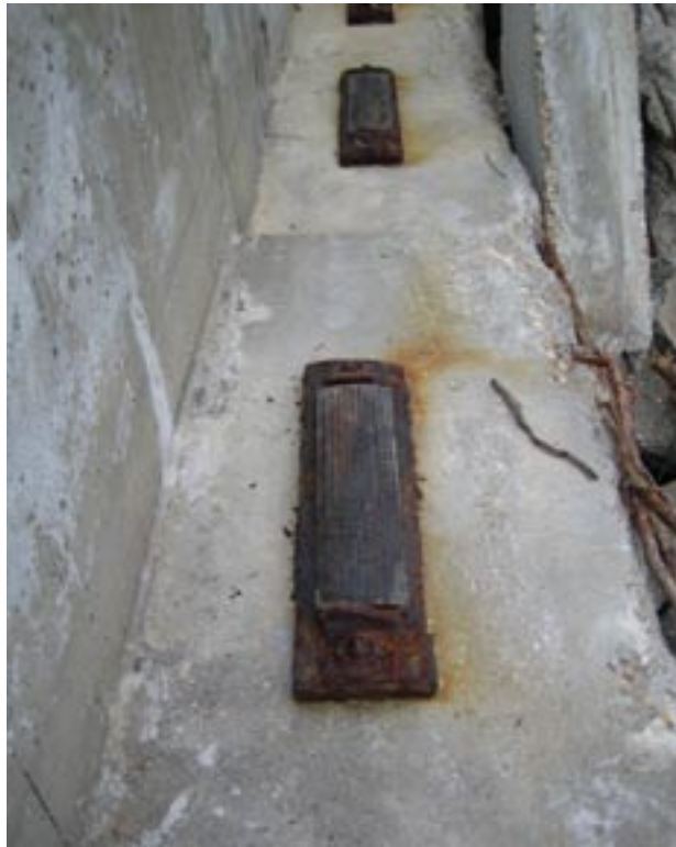
Figure 4.3 Biloxi Bay Bridge Bearings
