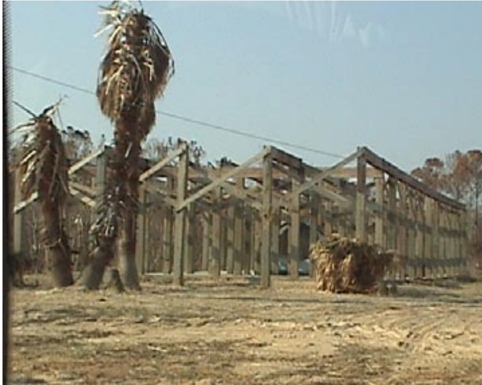
Figure 4.38. Survived Wood Pier System
