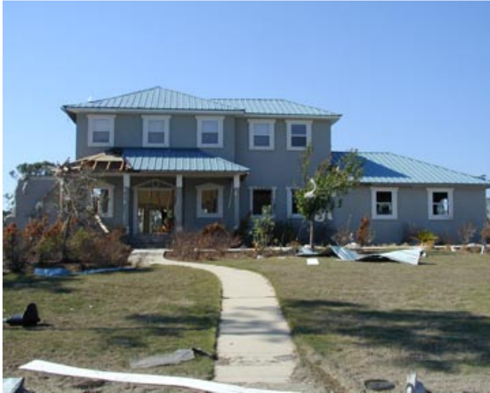
Figure 4.42. Survived SIP House with Wood Roof Damage
