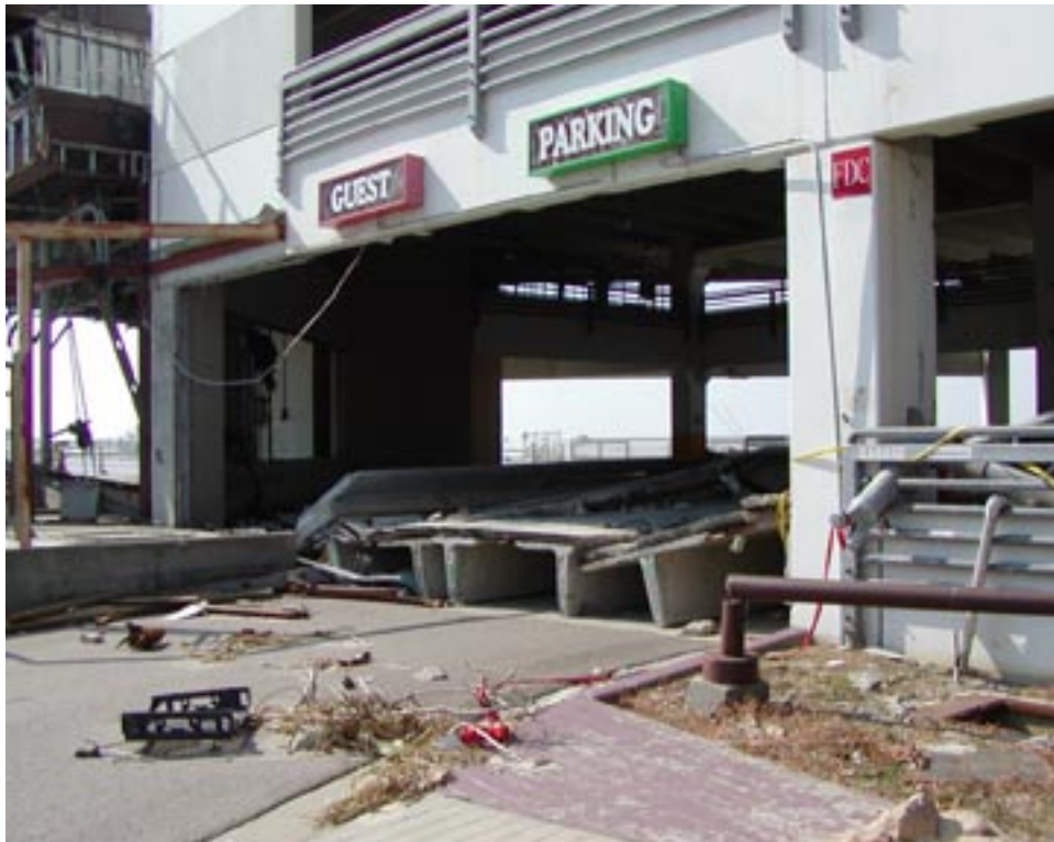
Figure 4.21. Failed PC Parking Structure
