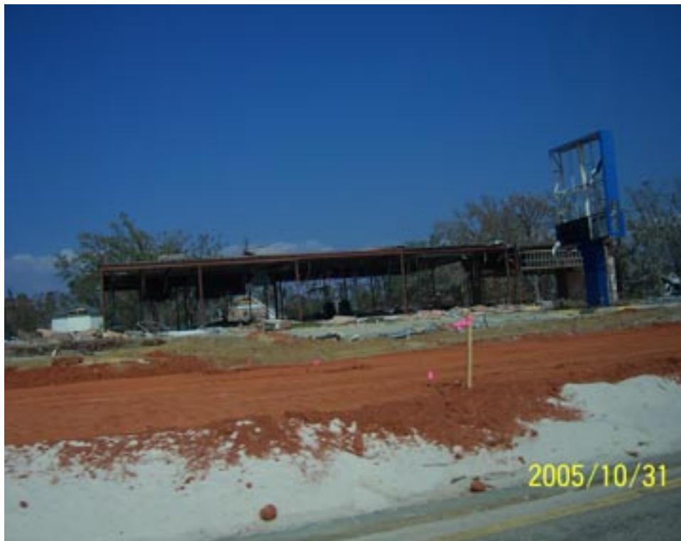
Figure 4.25 Survived Steel Frame
