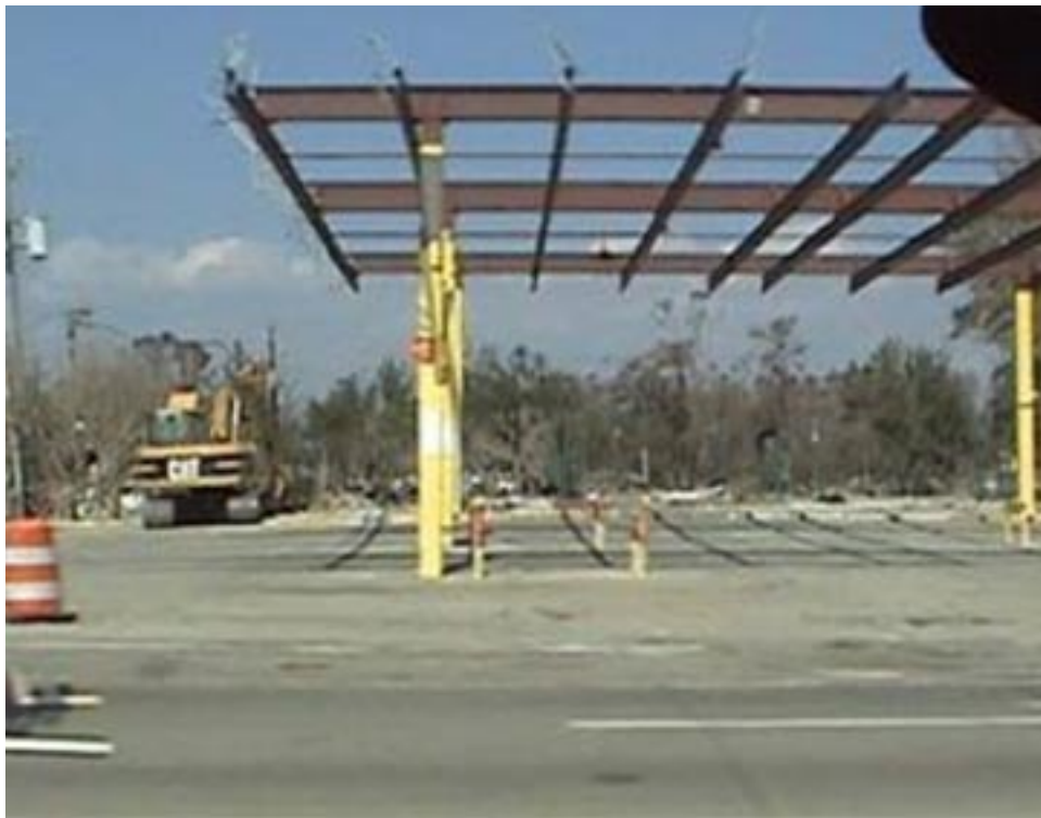
Figure 4.27 Survived Steel Frame
