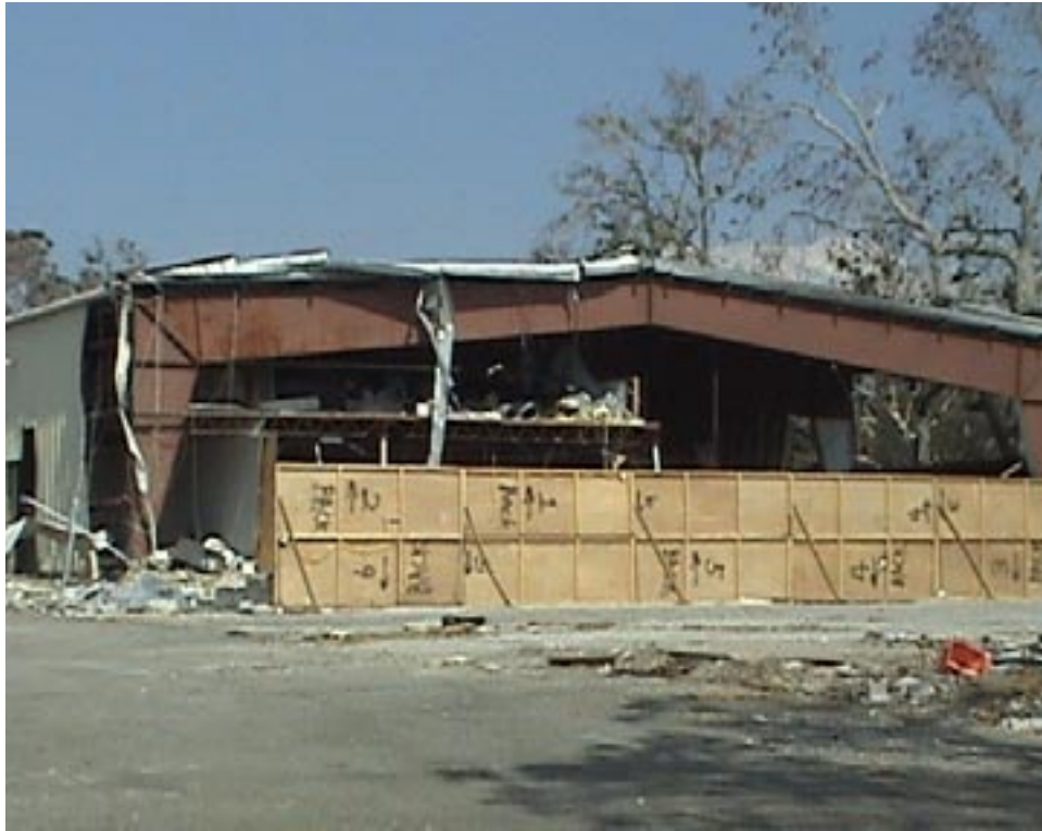
Figure 4.26 Survived Steel Frame
