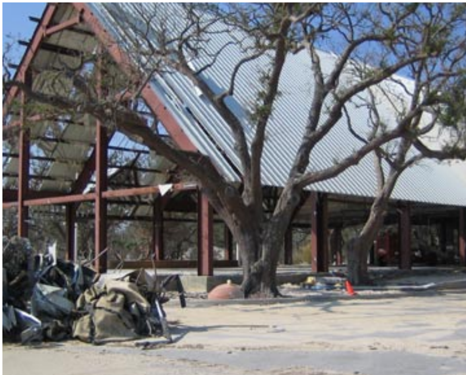
Figure 4.29 Survived Steel Frame
