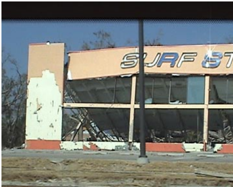
Figure 4.31 Failed Steel Frame with Open-Web Joist Roof
