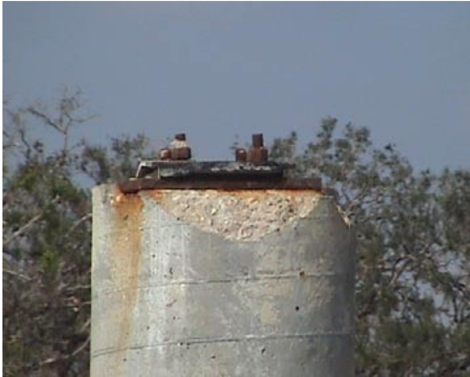
Figure 4.18. Failed PC Column Connection
