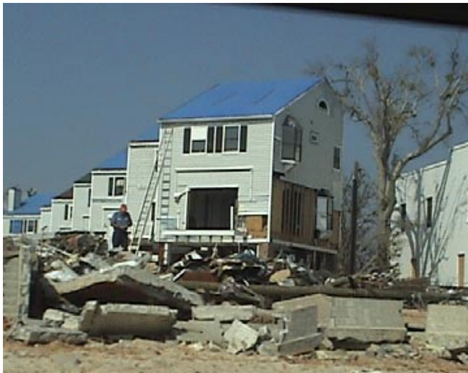
Figure 4.35 Siding Damage on Wood Building
