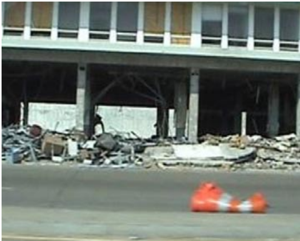
Figure 4.13 Survived RC Frame Structure
