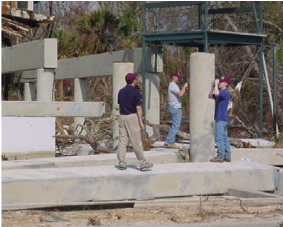
Figure 4.17. Failed PC Girder System
