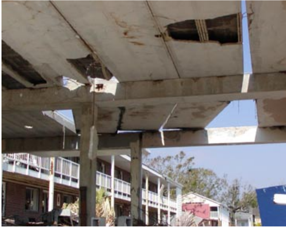
Figure 4.16. Failed PC Slabs Supported by RC Frame
