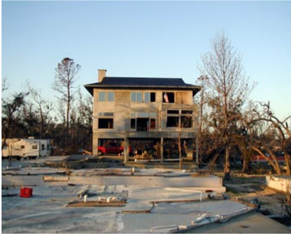
Figure 4.12. Survived RC Frame and Exterior Wall Structure.
