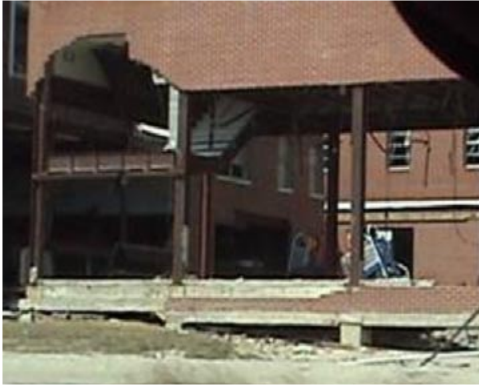
Figure 4.28 Survived Steel Frame
