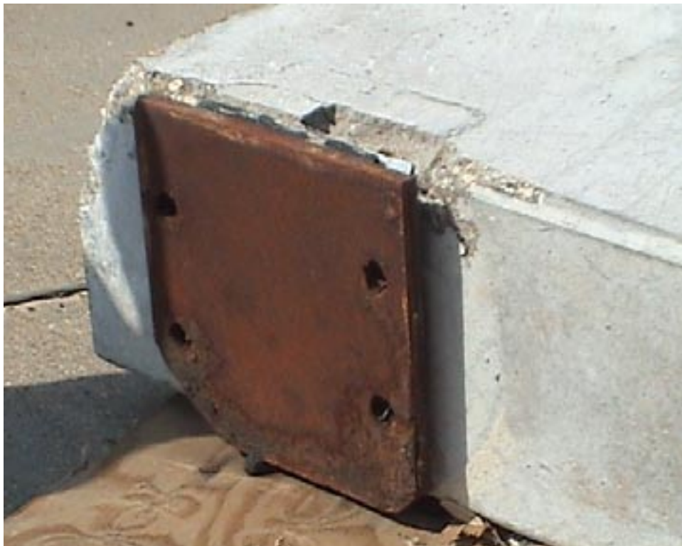
Figure 4.19. Failed PC Girder Connection
