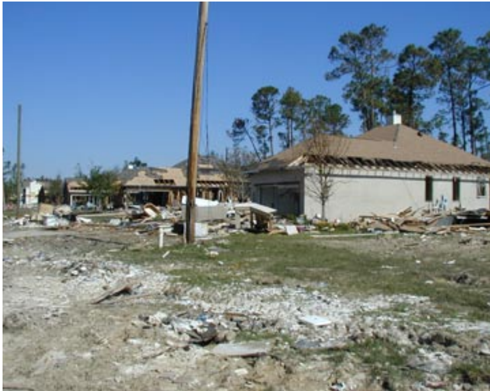
Figure 4.43. Survived SIP House, Severely Damaged Wood House in Background
