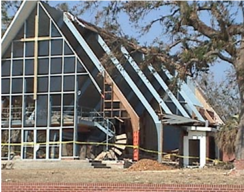
Figure 4.40. Survived Wood Glued-Laminated Structural Frame
