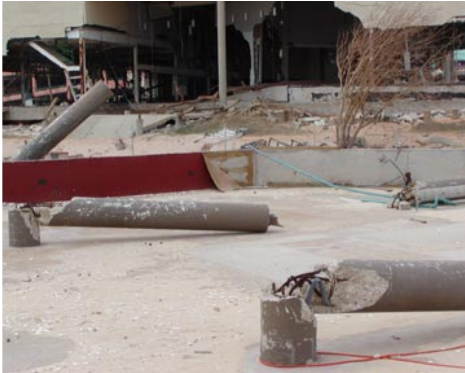
Figure 4.14 RC Failed Columns
