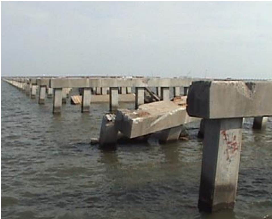
Figure 4.5 Pier Damage to Bay St. Louis Bridge
