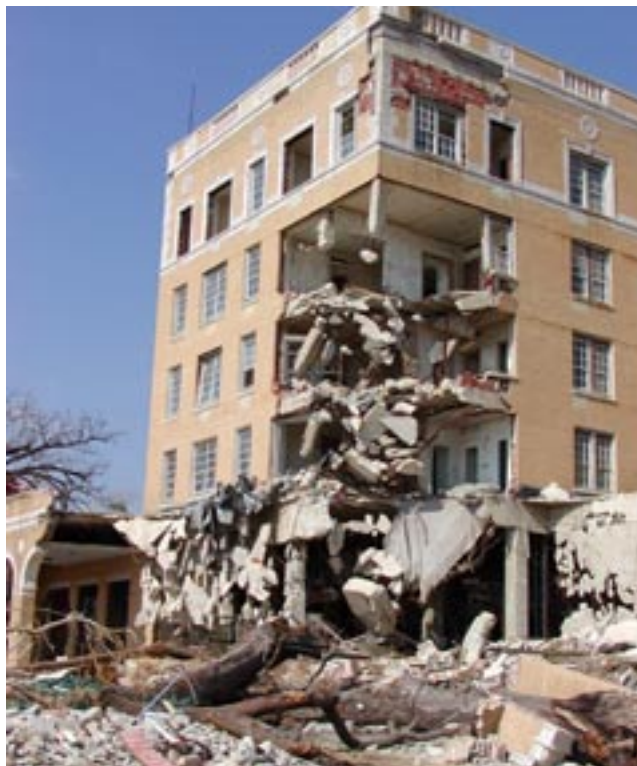
Figure 4.15. RC Frame Building Struck By Casio Boat
