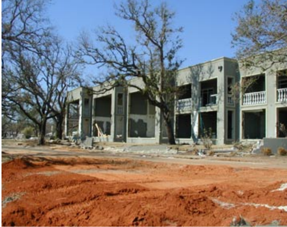
Figure 4.44. Survived SIP Structure
