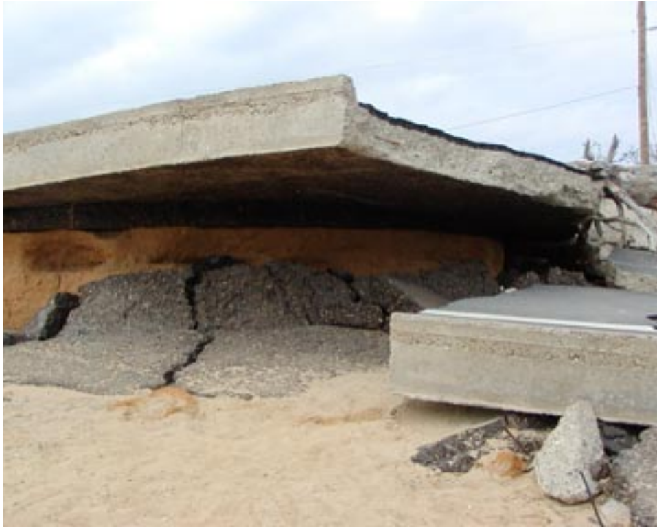
Figure 4.4. Biloxi Bay Bridge Road Undermining
