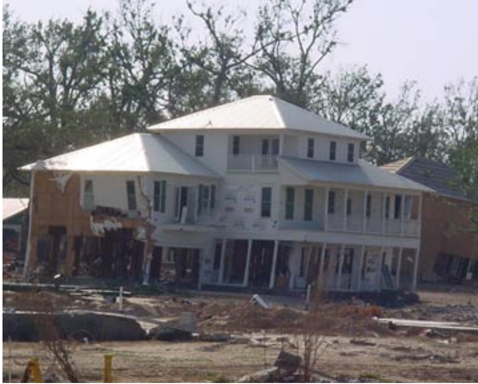
Figure 4.36 Side-Sway Failure in Wood House
