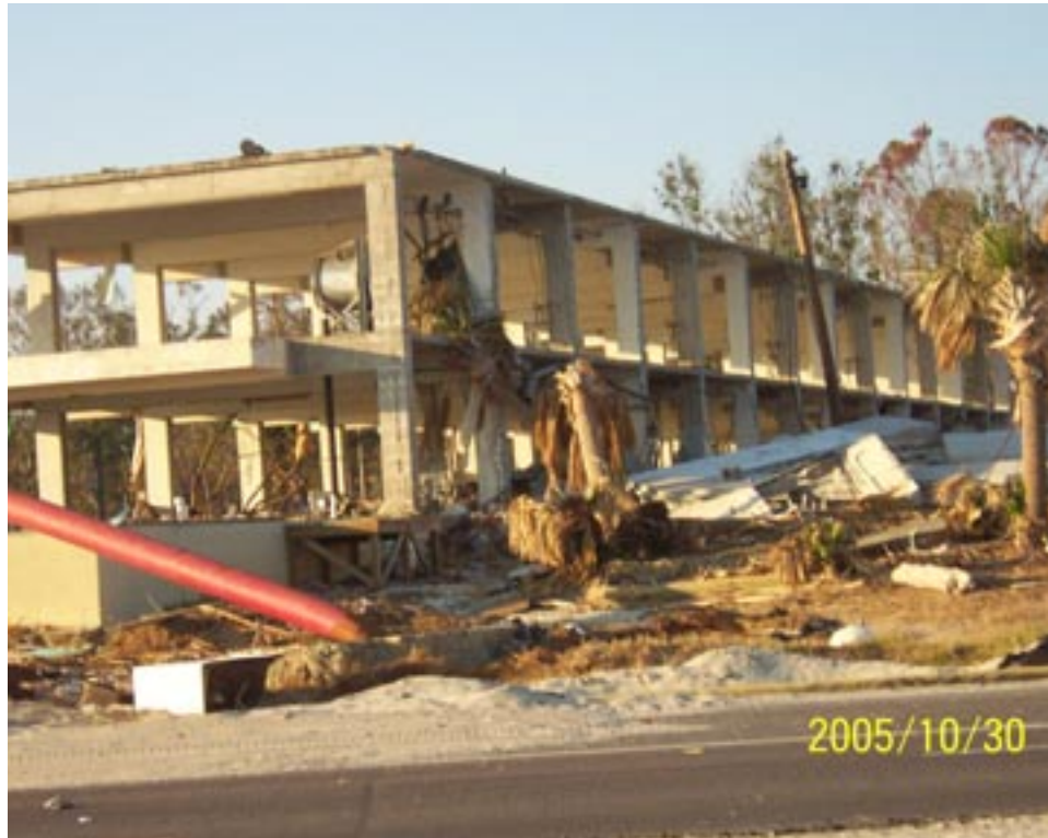
Figure 4.8 Survived RC Structural Frame
