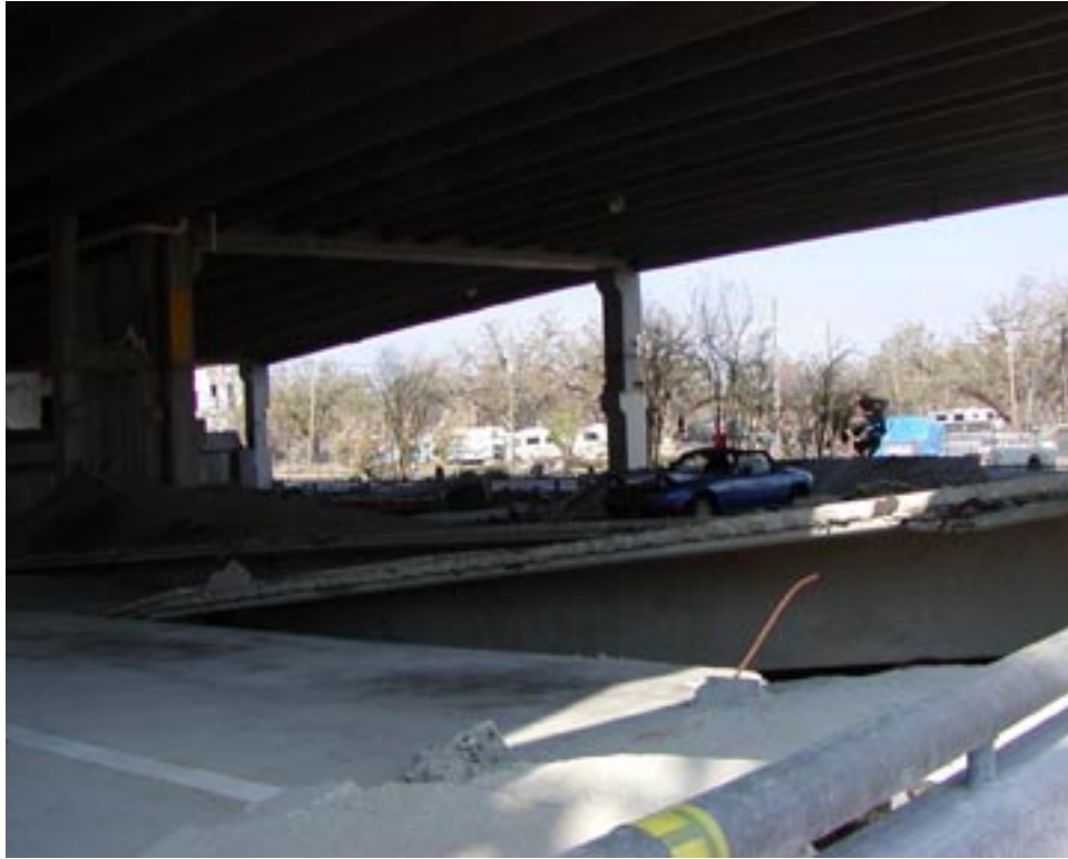
Figure 4.22. Failed PC Parking Structure
