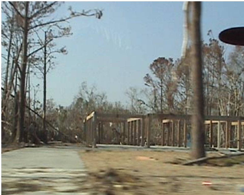
Figure 4.37. Survived Wood Pier System
