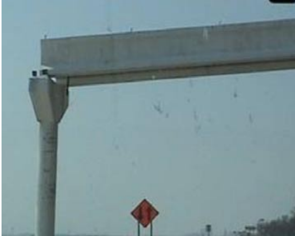
Figure 4.20. Failed PC Pedestrian Bridge
