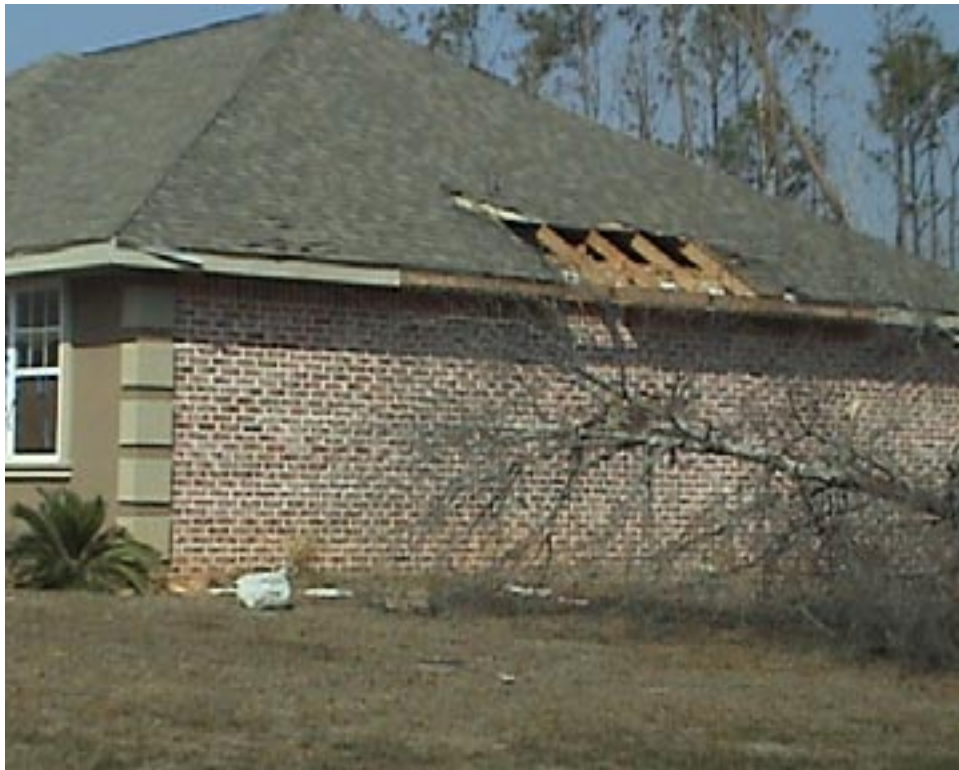
Figure 4.33 Roof Failure on Wood House
