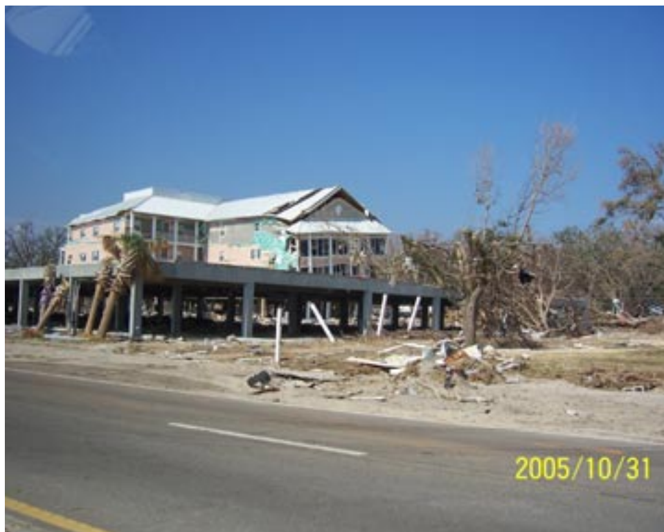
Figure 4.9 Survived RC Structural Frame that Supported Wood Superstructure
