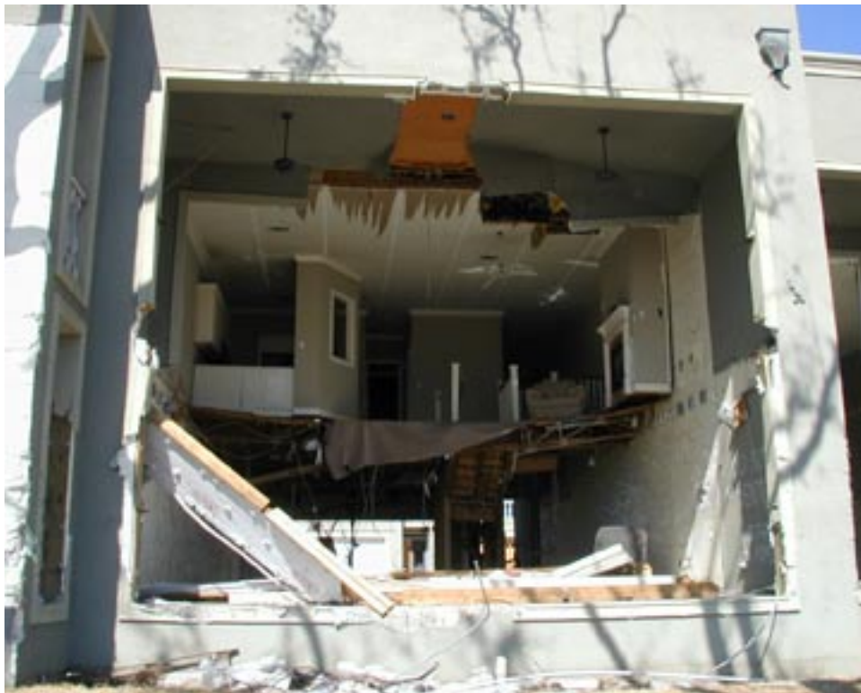
Figure 4.45. Survived SIP Structure with Destroyed Wood Floor
