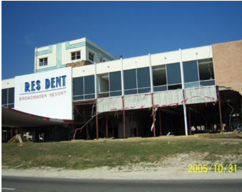
Figure 4.24 Survived Steel Frame
