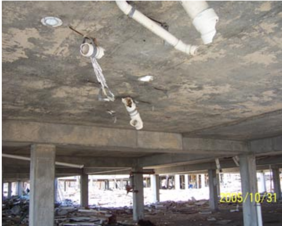
Figure 4.10 Close-Up of RC Structural Frame in Fig 4.12. Note no visible cracks or any other apparent structural damage.
