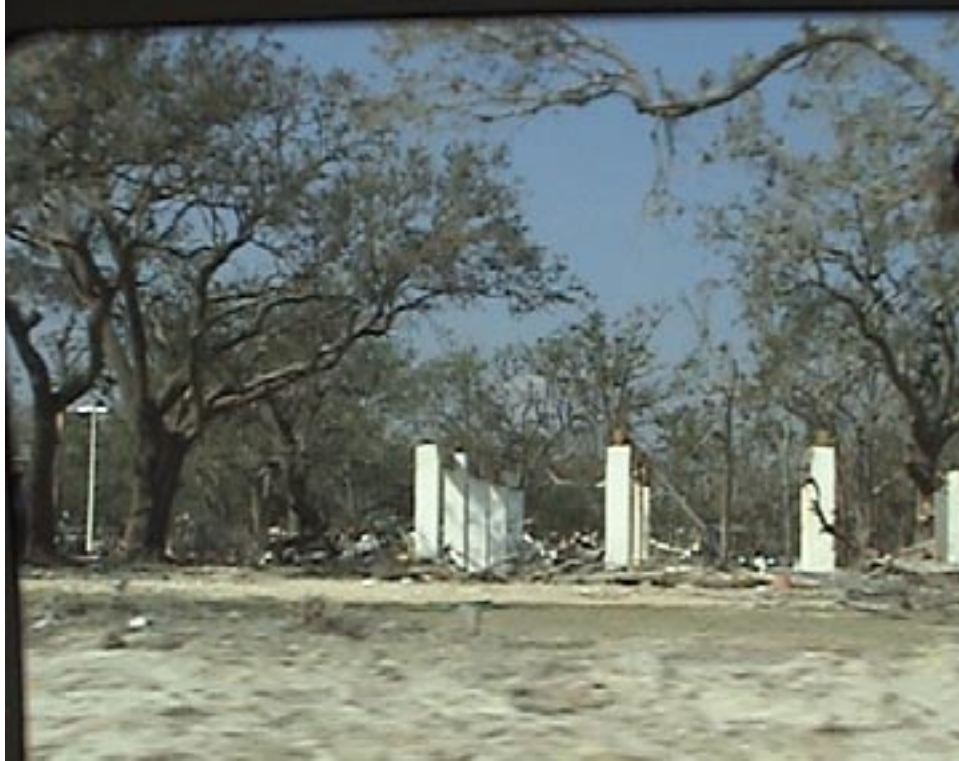
Figure 4.32 Typical Remains of Wood Structure--Superstructure Completely Destroyed
