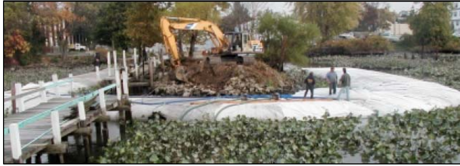
Figure 1.9. AquaDam® Units Used for Pier Construction
