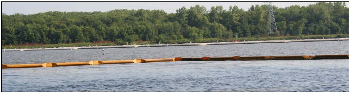
Figure 3.34. Turbidity Curtain Used During Peoria Island Construction
