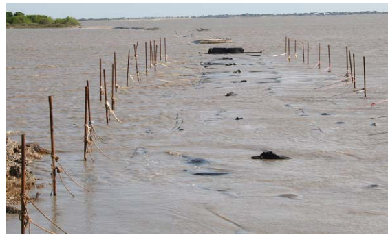
(b) Photo of Alignment Poles Connected to Handling Straps
