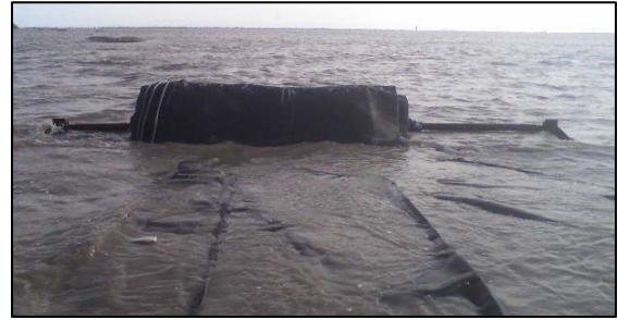
(b) Geotextile Tube on Pole Being Deployed
