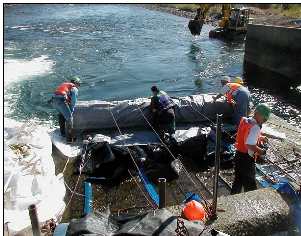
Figure 6.4. Ropes Used to Deploy Large AquaDam ® Units
