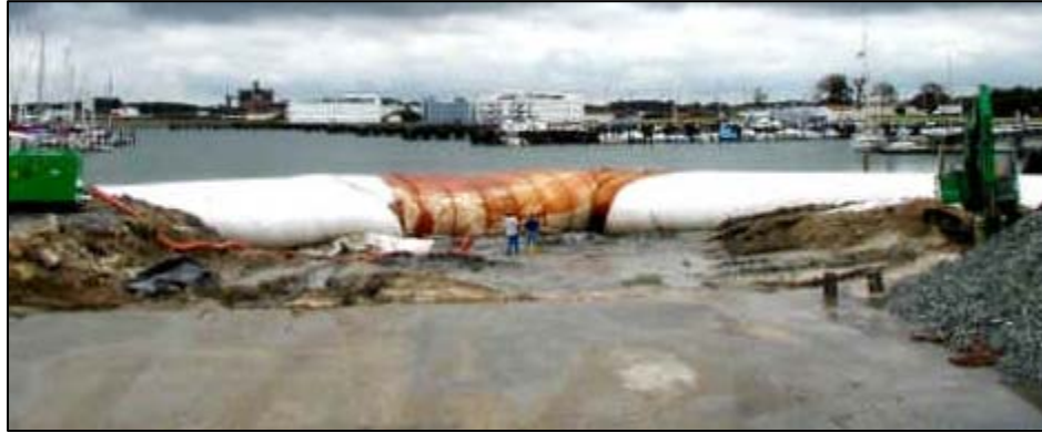
Figure 1.5. SPIRAL® Geotextile Tube Units Restraining Atlantic Coast Waters
