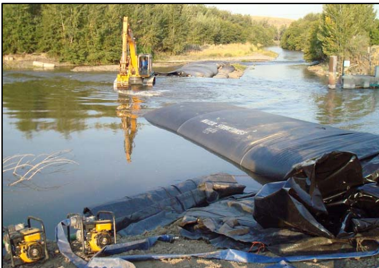
(a) Diverting Umatilla River
