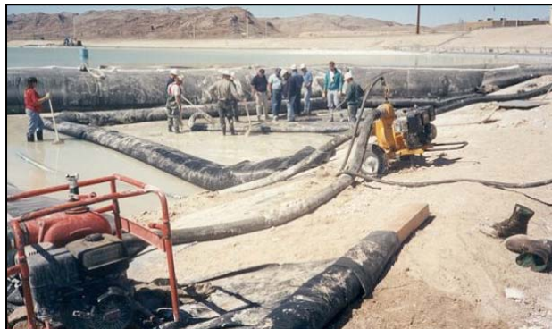
Figure 1.11. AquaDam® Units Used for Pond Liner Repair
