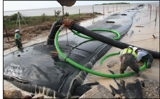
(b) Filling Geotextile and Anchor Tubes
