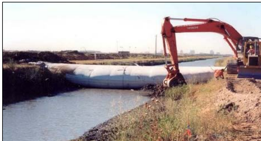
Figure 1.4. Temporary Blocking of Waterway
