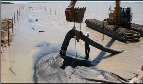
(a) Filling Geotextile Tube
