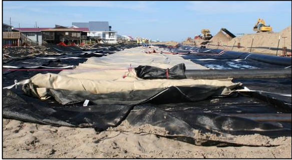
(a) Placed and Ready for Filling
