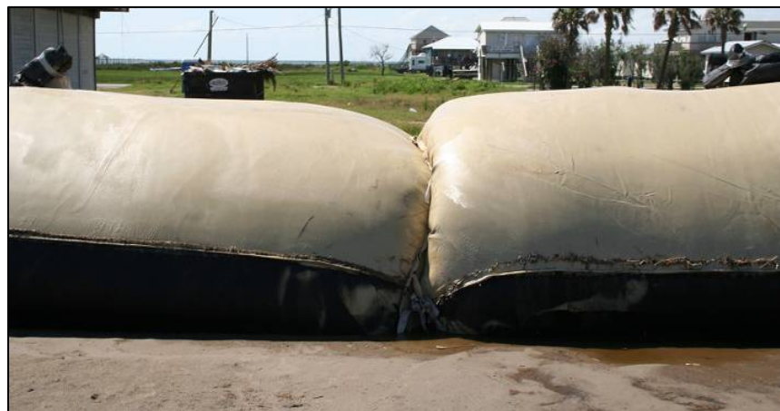
Figure 3.26. Ends of Two Geotextile Tubes After Filling
