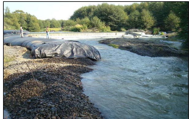
(b) Flow Diverted to One Side of the Weir
