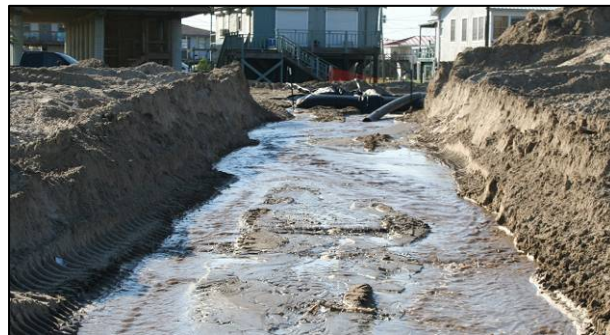
Figure 3.24. Trench Capturing Water Escaping Tubes During Filling
