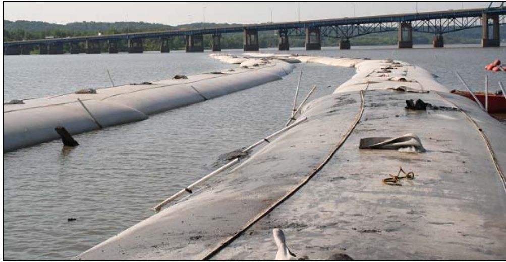
Figure 3.33. Geotextile Tubes Placed at Peoria Island
