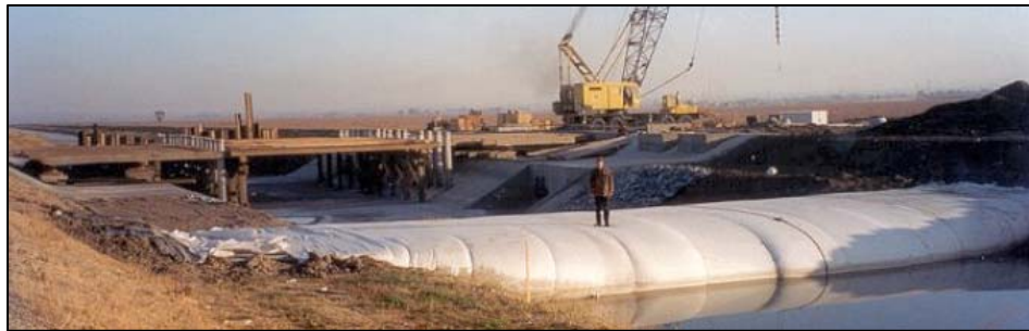
Figure 1.10. AquaDam® Units Used for Bridge Pier Construction
