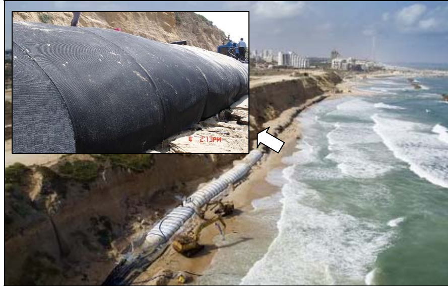
Figure 1.2. Bank Protection in Israel using Conveyor Belt Armor Cover
