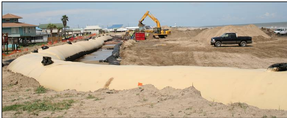
Figure 3.23. Curved Portion of Geotextile Tube Wall
