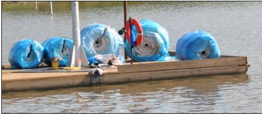
Figure 3.28. Peoria Island Geotextile Tubes Packaged and Awaiting Placement
