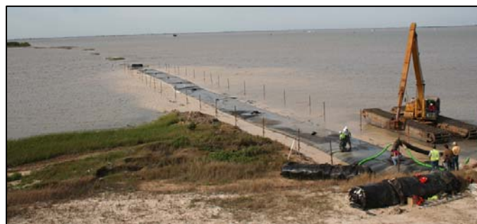
Figure 3.11. View of Matagorda Ship Channel Geotextile Tube Wall from Reclaimed Land
