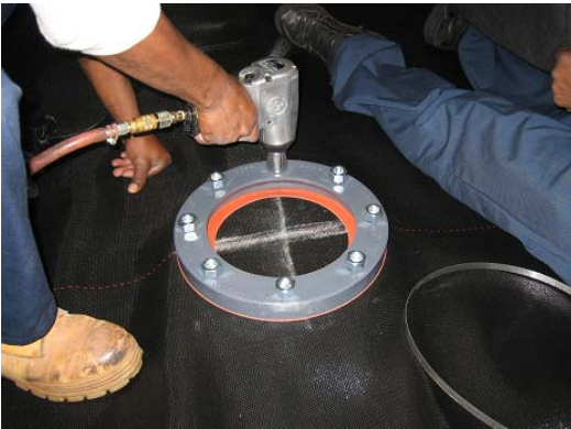
(c) Inserting Fill Ports
