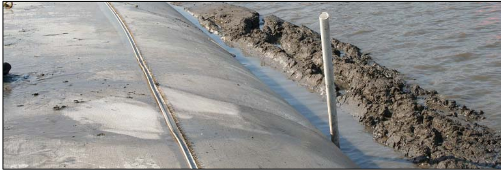
Figure 3.29. Settlement of Geotextile Tube
