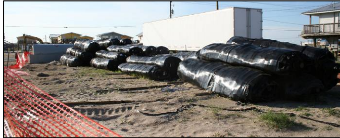
Figure 3.20. Geotextile Tubes at Grand Isle Awaiting Placement
