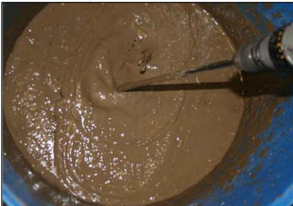
(f) Mixing of Stabilized Slurry (2 of 2)
