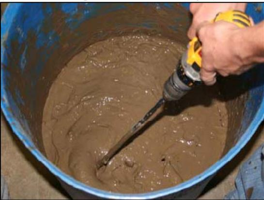
(e) Mixing of Stabilized Slurry (1 of 2)
