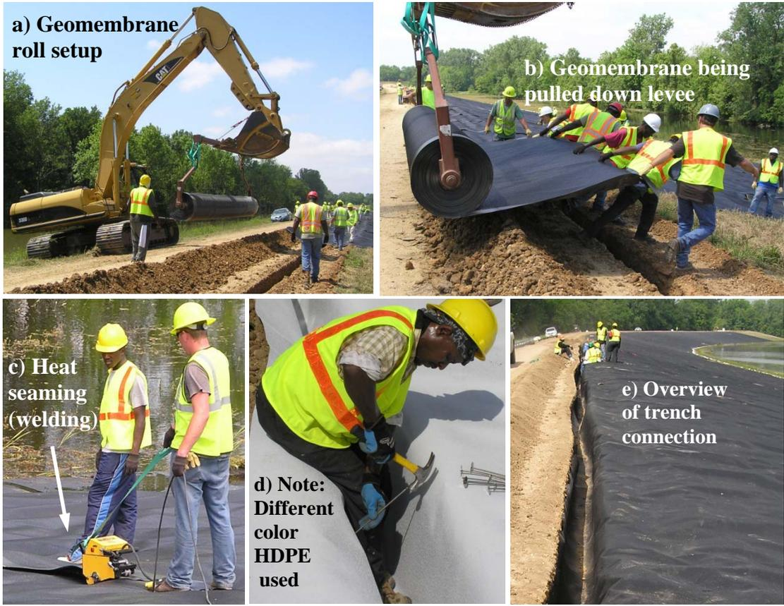
**Figure 3.4. Overview of Levee Protection Installation**
