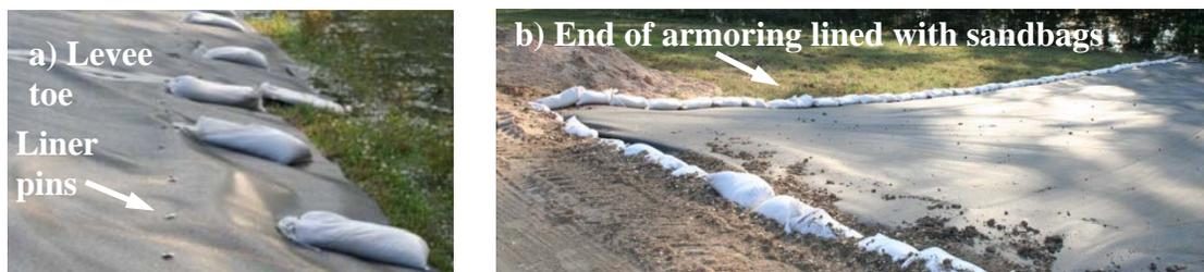
**Figure 3.7. Pinned Toe of Geomembrane**
