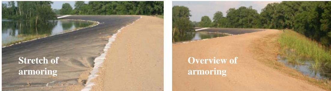
**Figure 3.2. Geomembrane Armoring of Landward Side of Backwater Levee**
