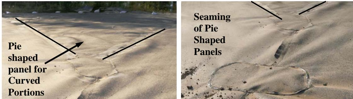
**Figure 3.8. Panel Installation in Curve Portions of Protection**
