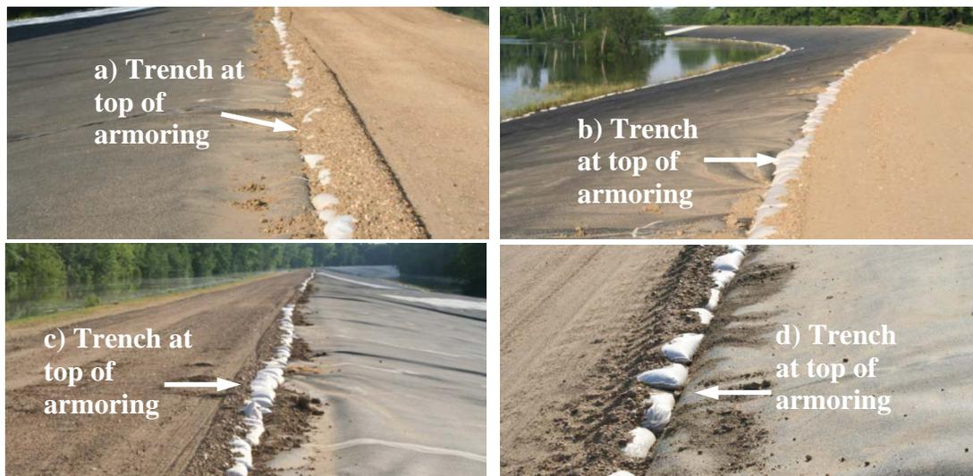
**Figure 3.6. Trench of Armored Levee Protection**
