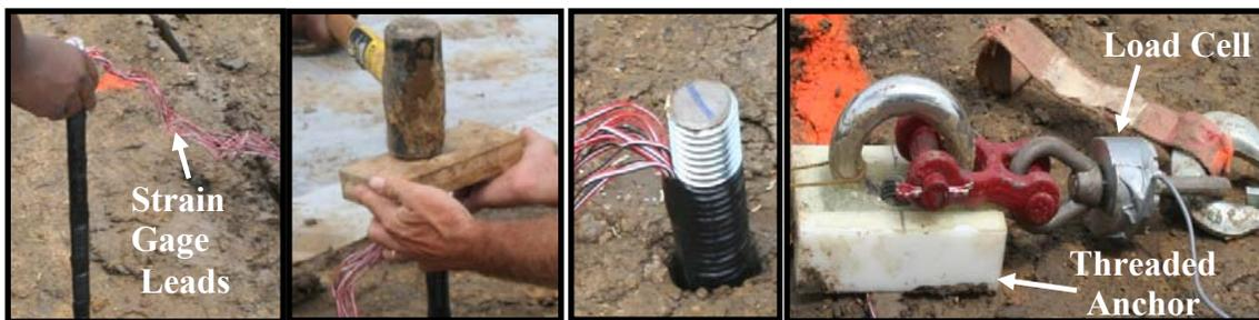
**Figure 4.10. Installation of 0.6 m Threaded Bar Anchor**
