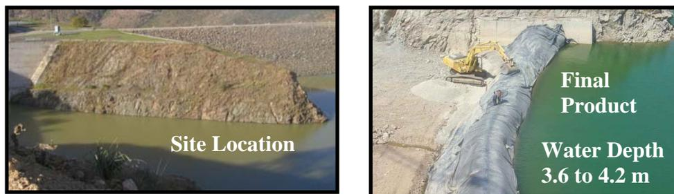
Figure 12. Construction of Temporary Dam in Morocco Using Geotube® Units
