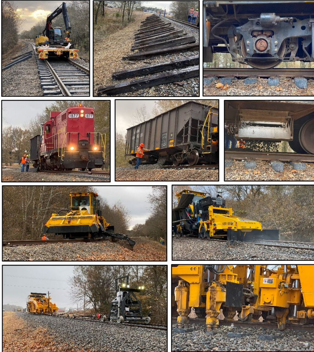
Figure 3.4. Photos of McAlester test sections under construction
