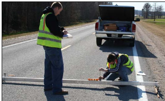
Figure 3.14. Manual Rut Measurements
