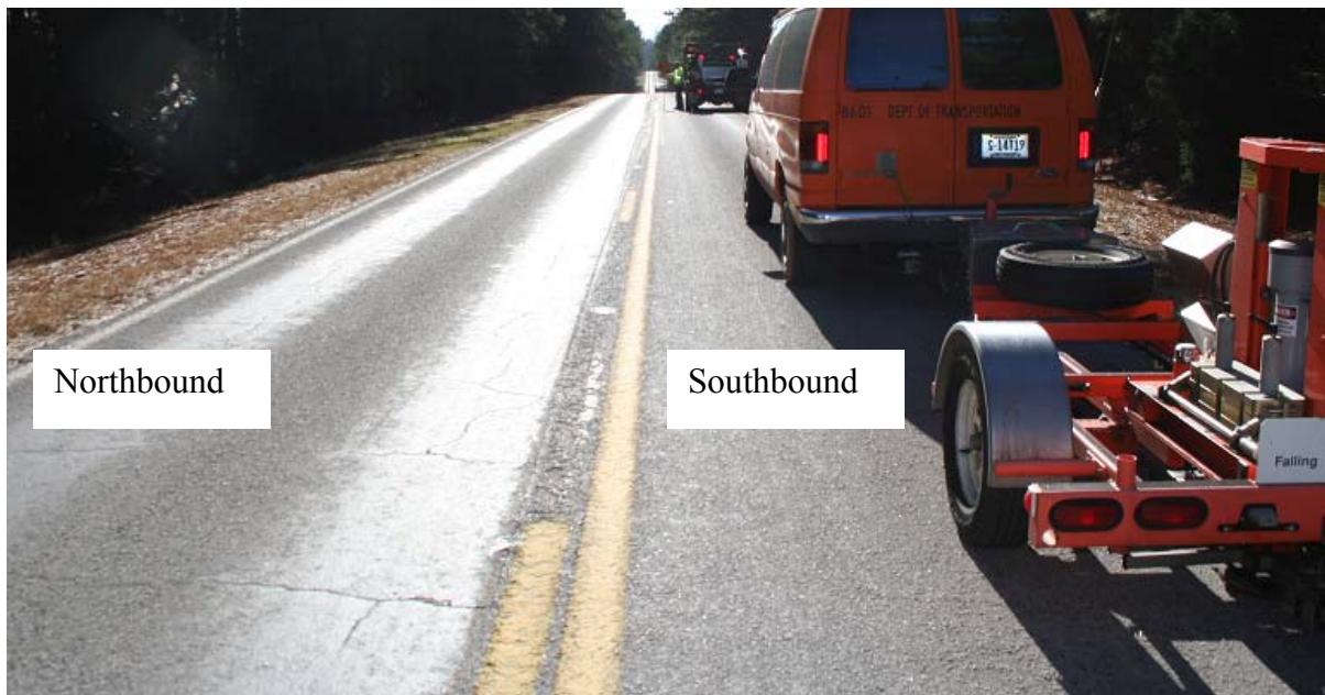
(b) Relative Bleeding/Flushing Photo 2 of 2
